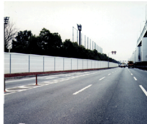
View of the soundproof highway walls coated with TiO 2 photocatalysts for the elimination of NO x . (Osaka, April 1999)
